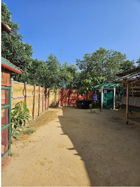
Fig. 12:., fencing around the Maiya School
