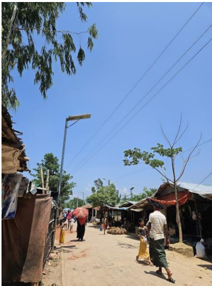
Fig 16: Main road in Camp 22, Unchiprang
