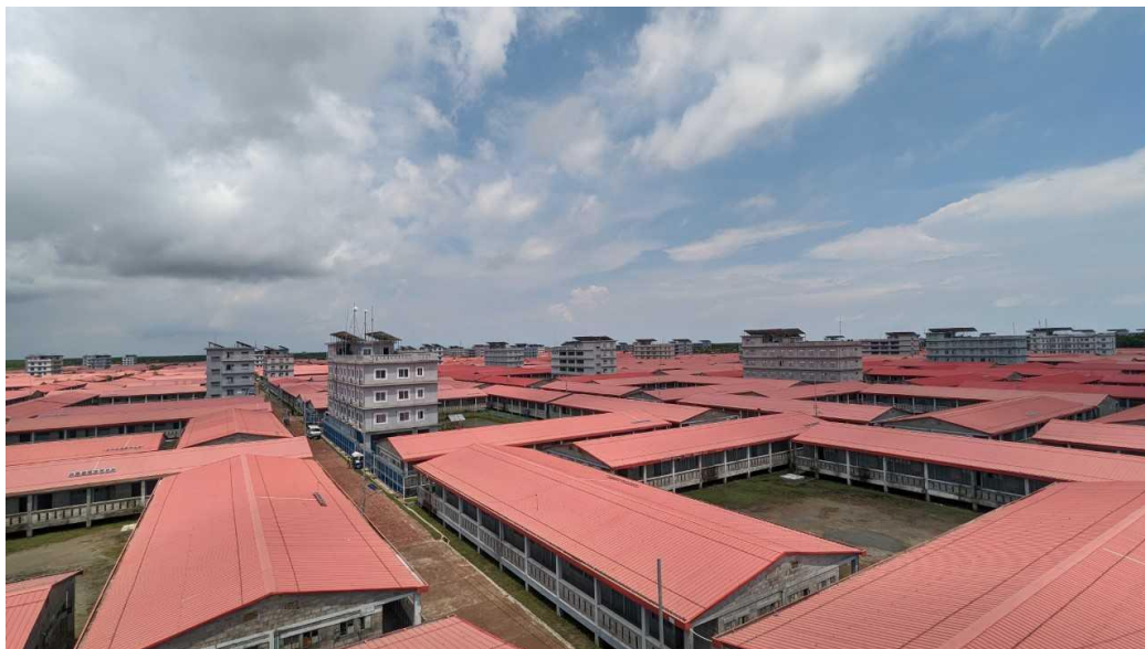
Fig. 4: Completed shelters in Bhasan Char, off the coast of Cox's Bazar (credit: Javed Kaisar)
